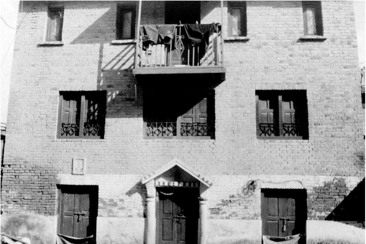
Figure 20 Pre-earthquake Newar house in Sankhu partially reconstructed since 2015 earthquake, December 2023.
